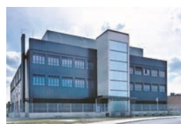
Germany Frankfurt 4 Data Center
