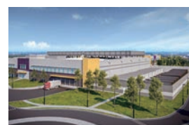
Virginia Ashburn 4 Data Center
